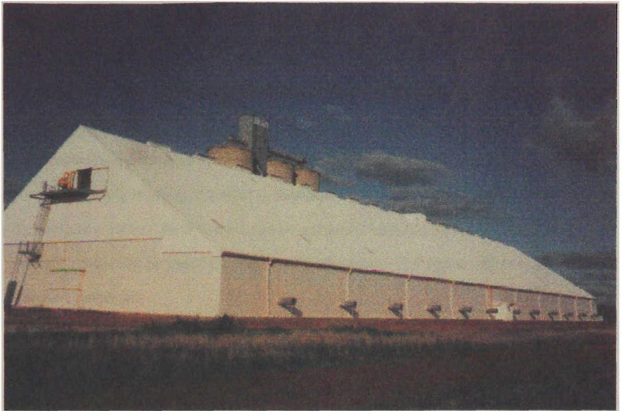
Fig. 4.10 - Large shed-type grain store showing aeration fans to which M c Bea Mobile Grain Coolers can be attached during the summer following harvest for chilling the stored grain Courtesy Graincorp Limited, New South Wales
