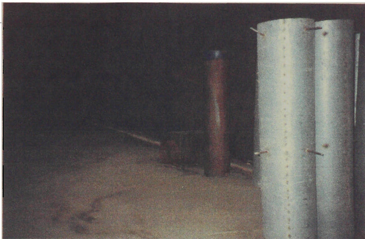
Fig. 4.8 - Perforated metal aeration ducting with strengthening cross bracing rods protruding to inhibit movement of the duct when placed horizontally on the floor.
