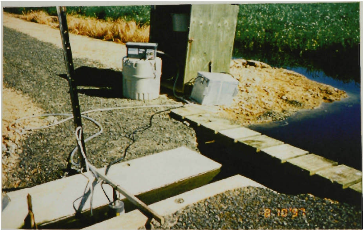
Figure 4.2 Rectangular Concrete Lined Outlet Structure
