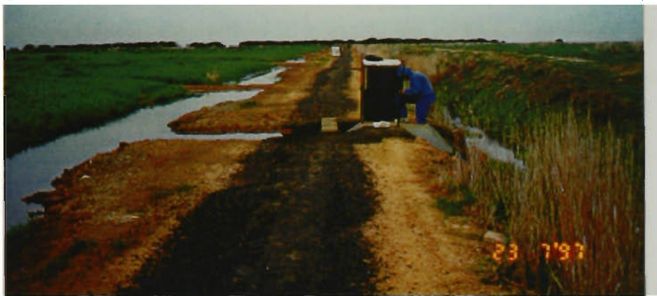
Figure 3.3 Grass Filtration Bays - Bay Outlets - Common Drainage Channel: (From Left to Right)
