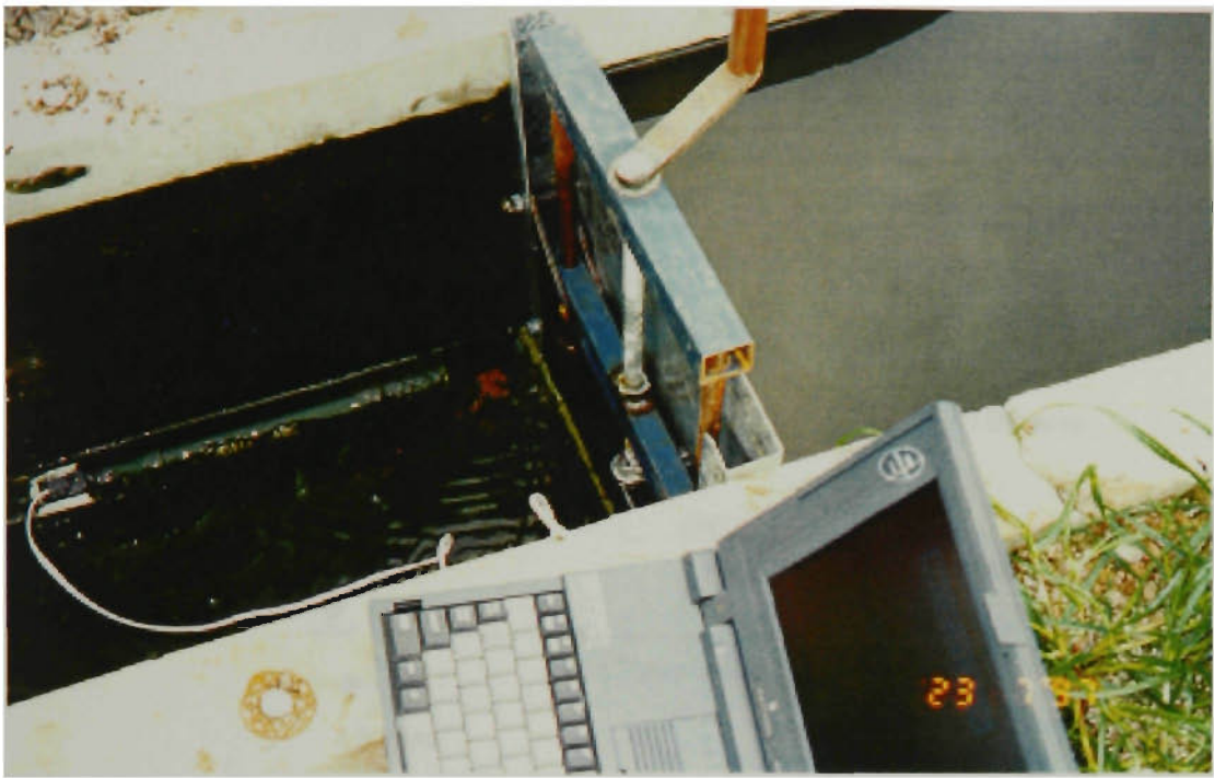
Figure 4.1 Rectangular Concrete Lined Inlet Structure with Depth Logger Installed Inside
