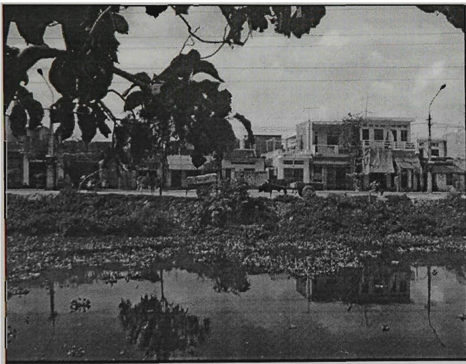
Plate 6. The Kim Ngừ Drain upstream from Thanh Trì during the dry season showing low flow rate, high nutrient load and evidence of eutrophication.
