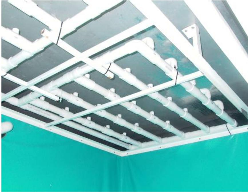
**Figure 6.10.** A view of the water distribution system from below. It is supported by a light metal frame.
