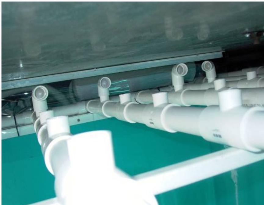
**Figure 6.9.** Water distribution system in the roof of the shipping container. Water goes out of the inverted tee-pieces and the pipe elbows.
