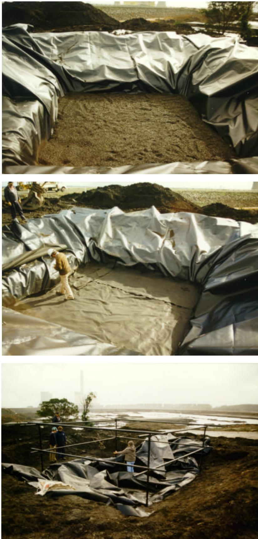
Figure A3.2 - Coarse drainage layer; bitton cloth, steel framework.
