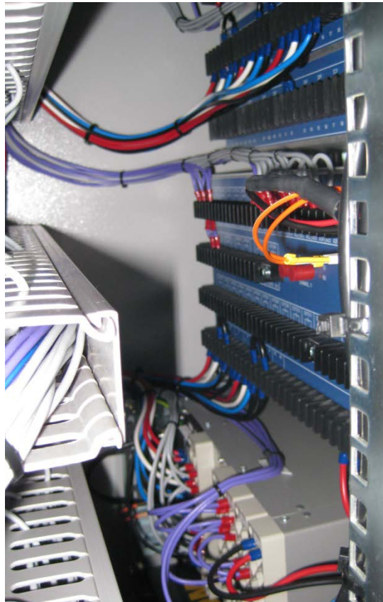
Figure A.42: IED wiring connections
