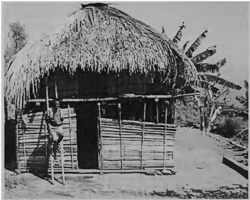
Photo 8. Maize storage in Maubara – kitchen with maize storage area above, accessible by ladder
