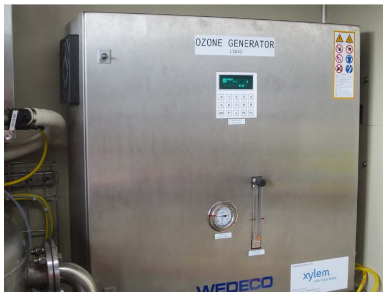
Figure x – Ozone generator, ozone system, Section 1
