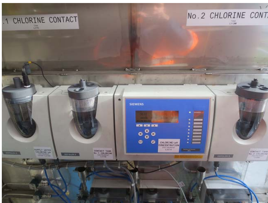
Figure x – Chlorine analysers, Chlorine Dosing system, Section 3
