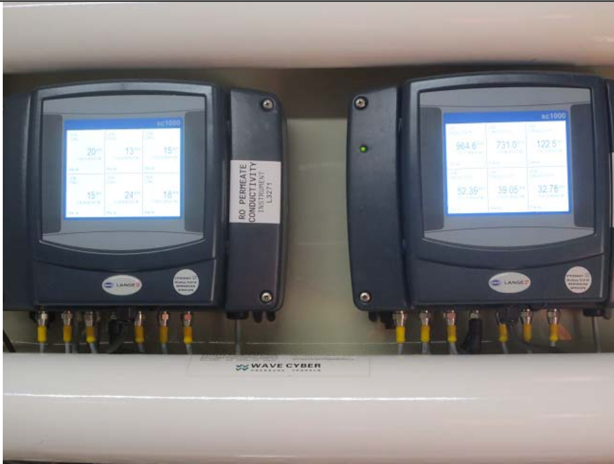
Figure x – Conductivity analysers, RO system, Section 2
