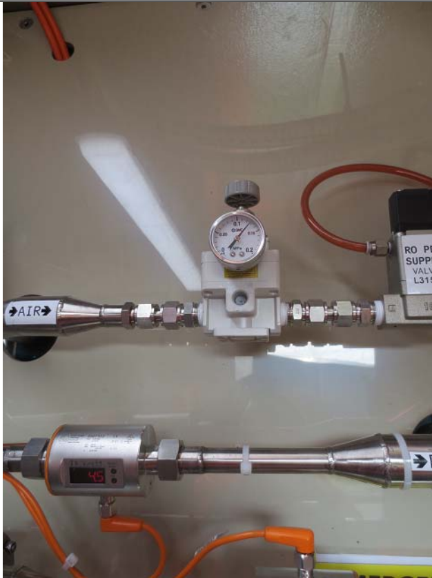
Figure x – Pressure indicator in RO system, Section 2
