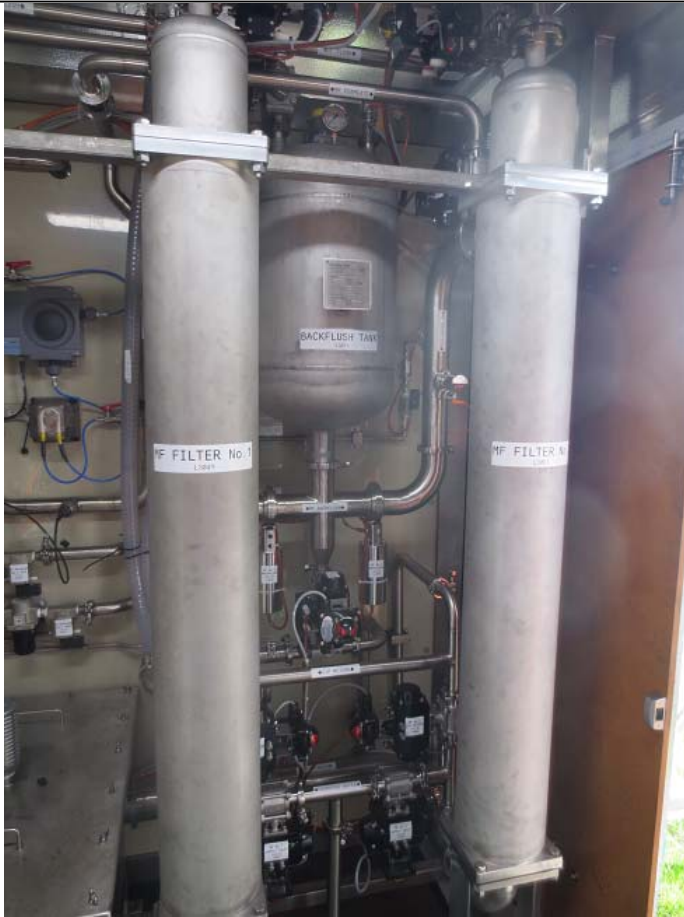
Figure x – MF Filters and back flush tank, MF, Section 1
