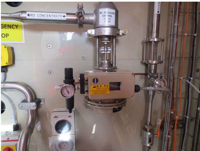
Figure x – Proportional flow valve, RO system, Section 2
