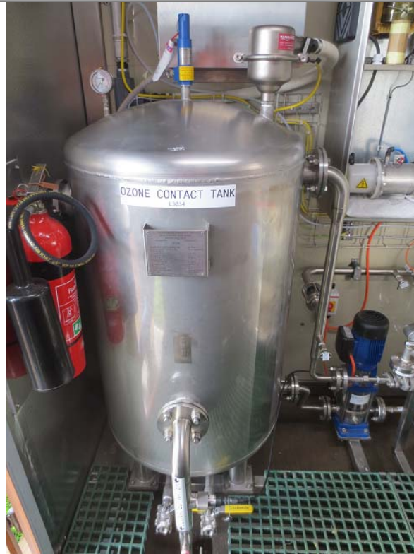
Figure x – Ozone contact tank, ozone system, Section 1
