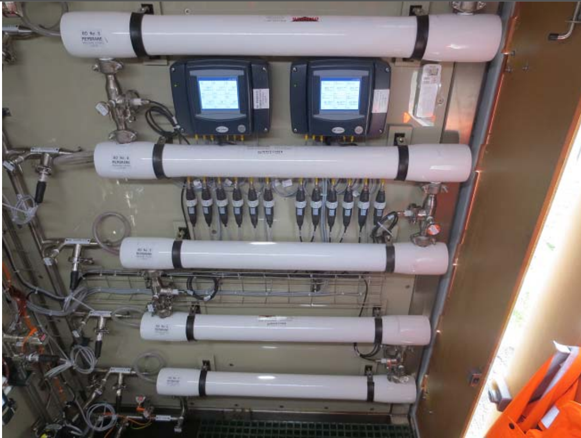
Figure x – RO pressure vessels, RO, Section 2
