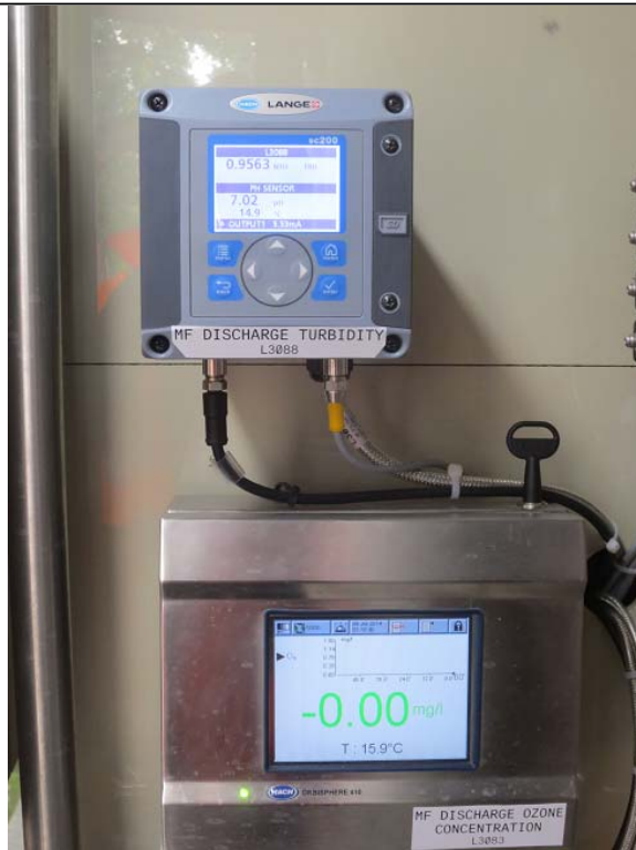
Figure x – Dual display for turbidity and pH transmitters (top), MF, Section 1
