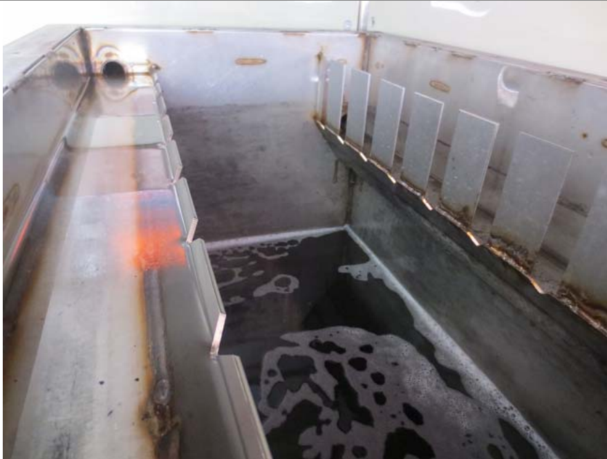
Figure x – BAC filter interior, BAC, Section 2. MF filtrate enters the BAC through the channel on the left. During back flushing, back flush water flows into the channel on the right and into the waste tank.
