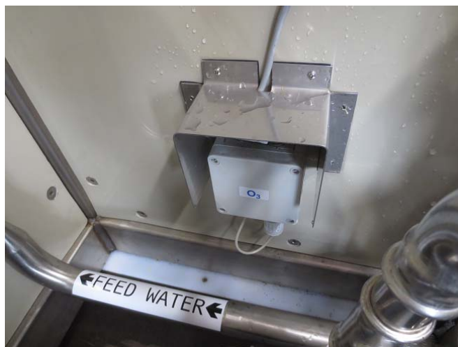
Figure x – Atmospheric ozone detector, Ozonation system, Section 1
