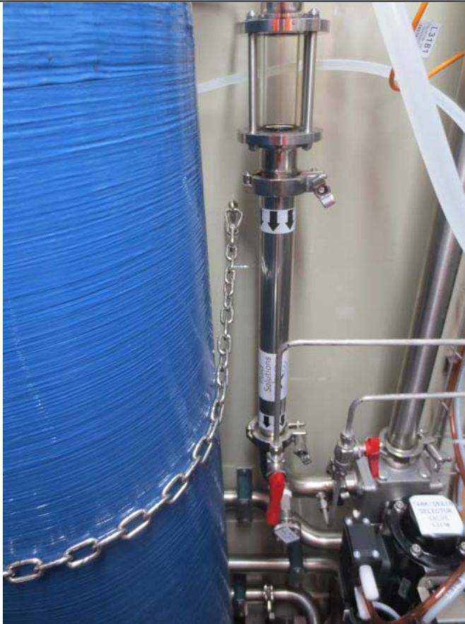
Figure x – Static mixer, Chlorine Dosing, Section 4
