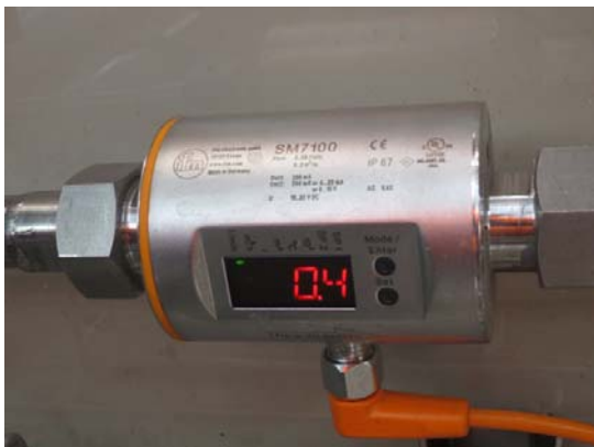
Figure x – Magnetic flowmeter used throughout AWTP
