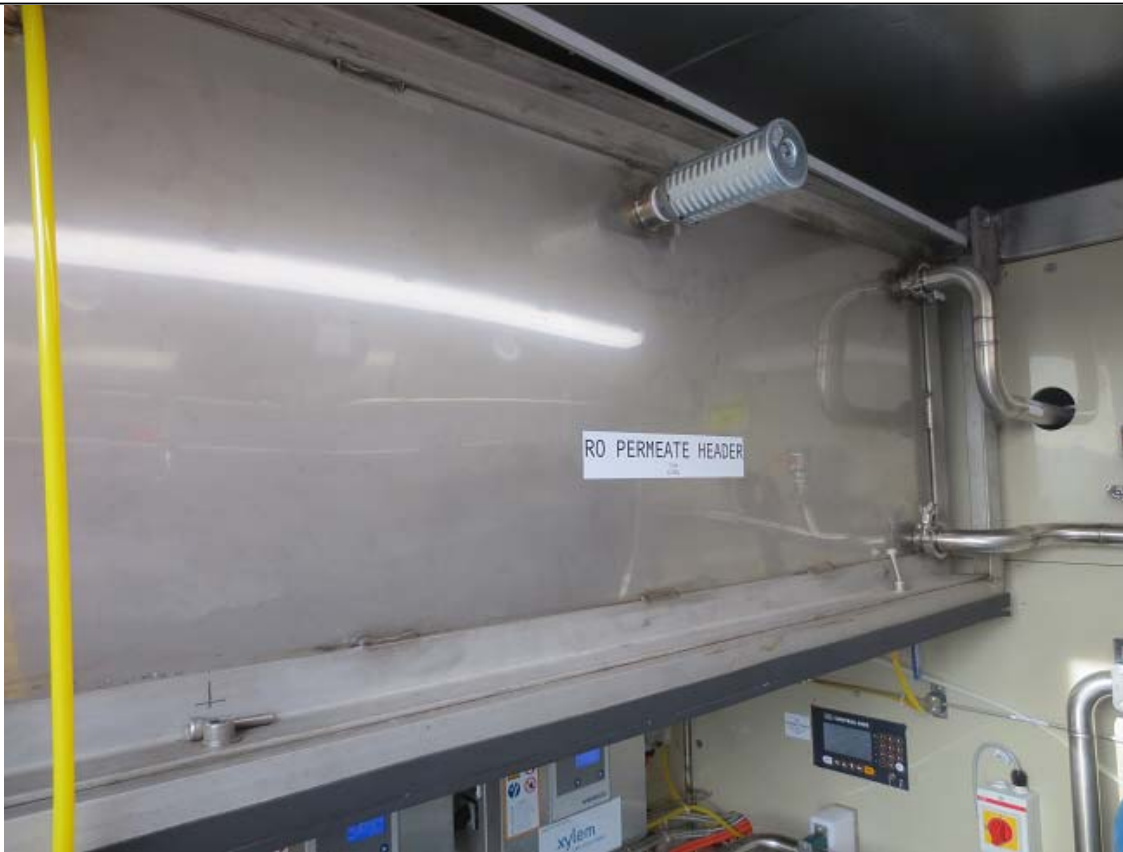
Figure x – RO permeate tank, RO, Section 3
