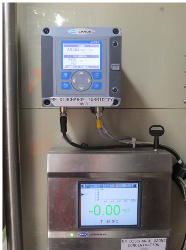
Figure x – Ozone Residual Analyser (bottom instrument), Ozone System, Section 1
