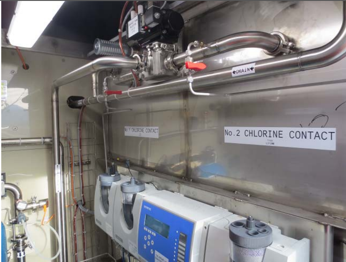
Figure x – Chlorine contact tanks and chlorine meters, Chlorine Dosing, Section 3
