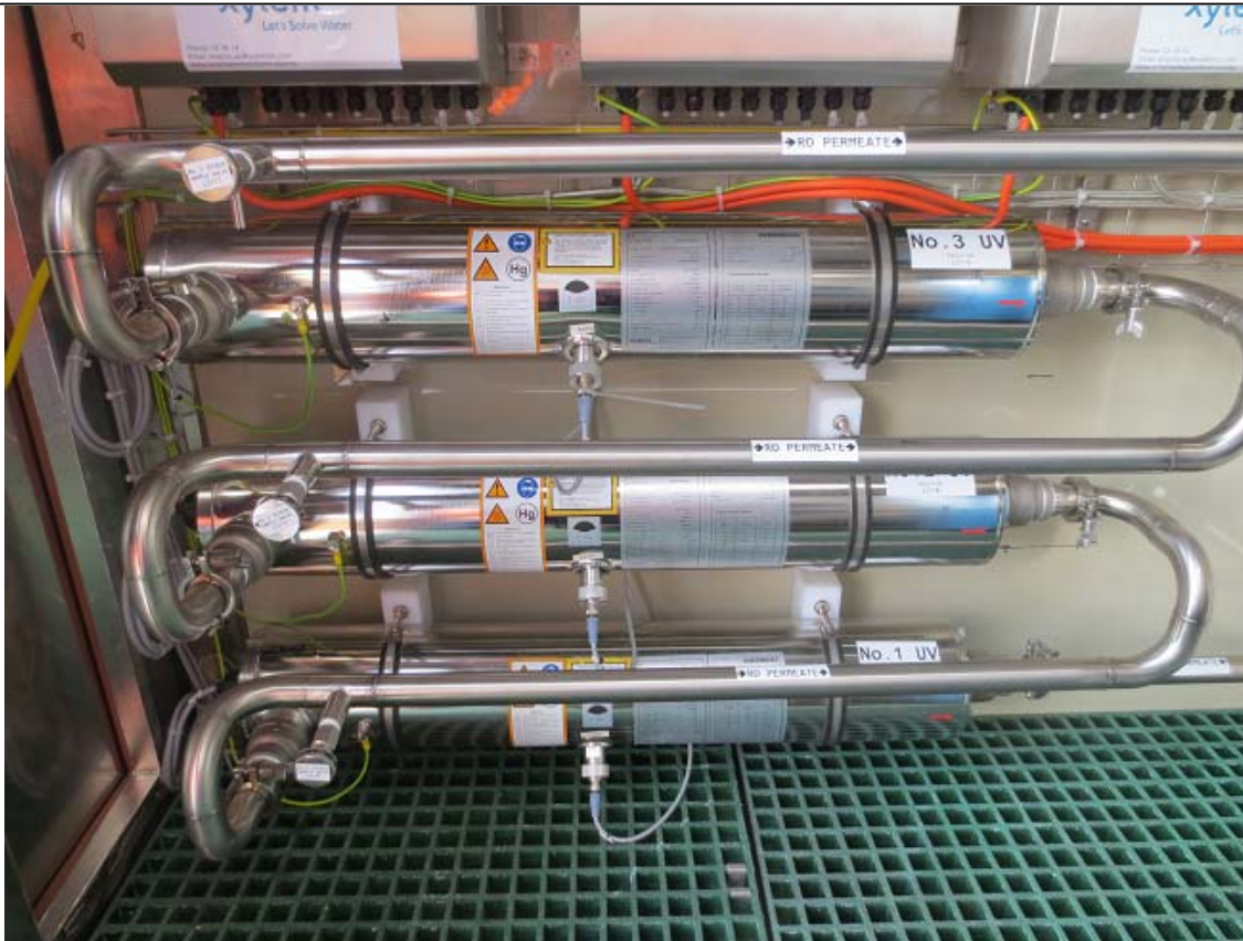
Figure x – UV reactors, UV, Section 3
