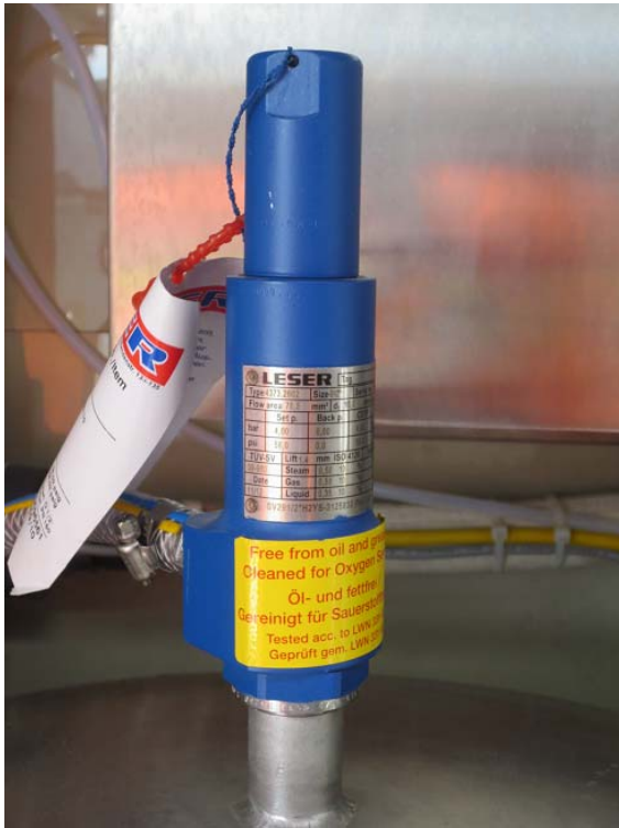
Figure x – pressure relief valve on ozone contact tank, Ozonation System, Section 1
