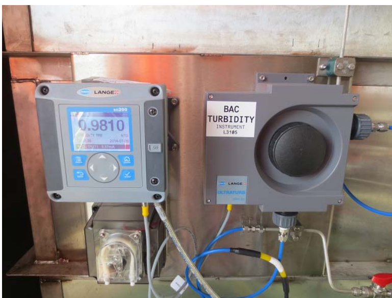
Figure x – Turbidity analyser, BAC filtrate line, Section 2
