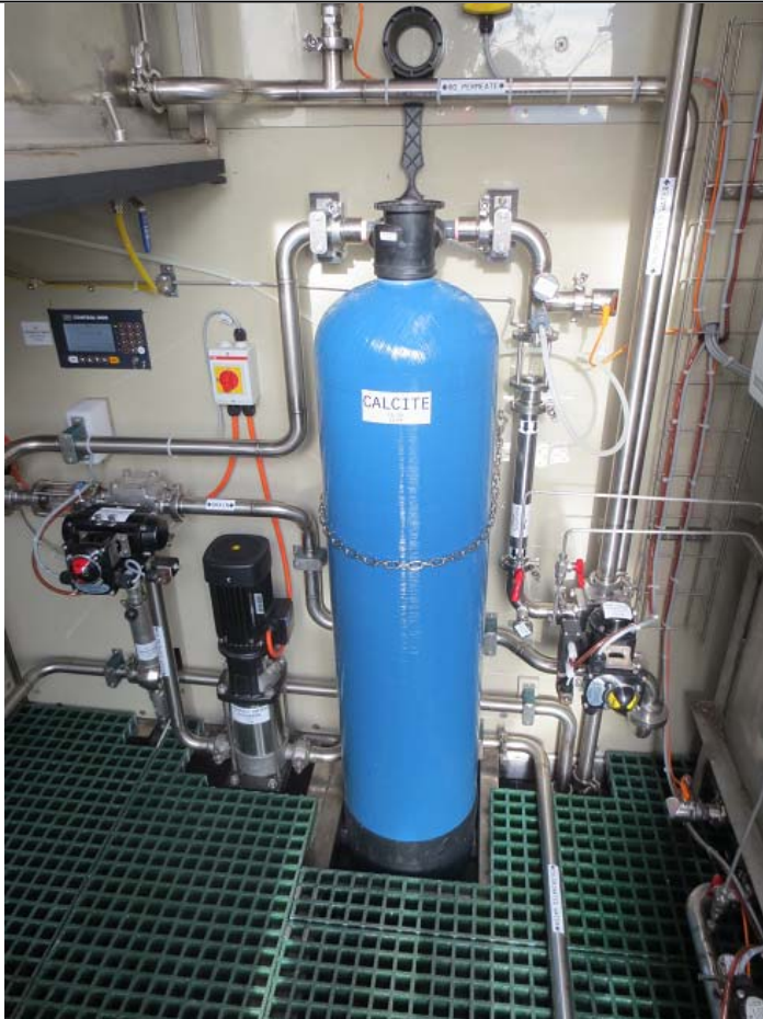
Figure x – Calcite contactor, Section 3
