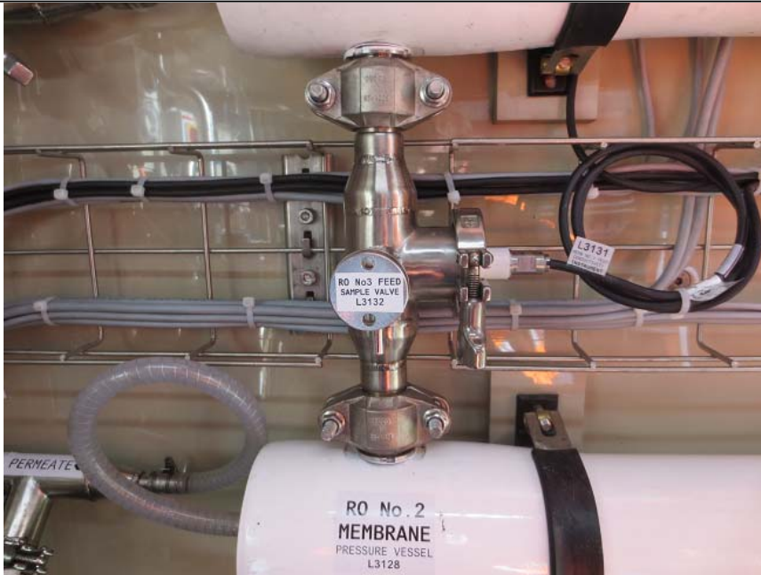
Figure x – Sample valve on RO concentrate line, RO system, Section 2
