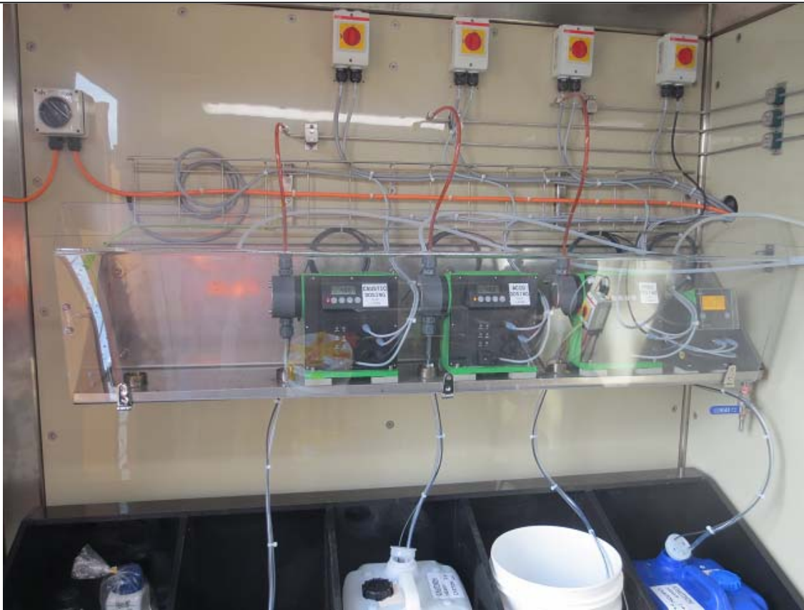
Figure x – Chemical bunds and dosing pumps, CIP, Section 4
