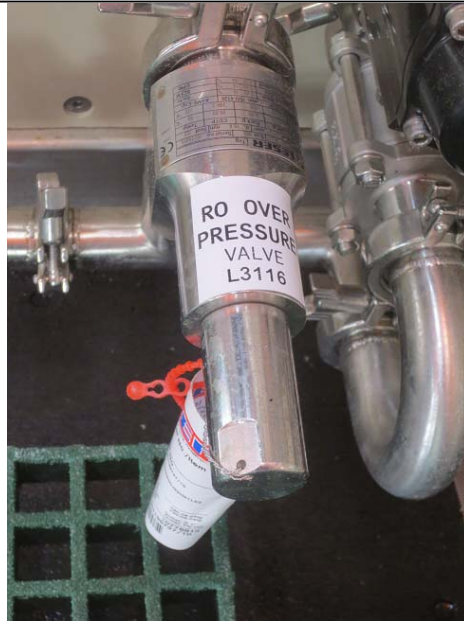
Figure x – RO pressure relief valve, RO system, Section 2
