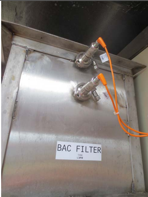
Figure x – Level switches, BAC, Section 2
