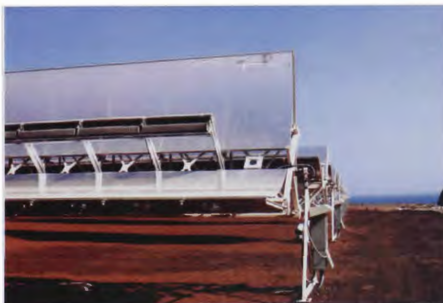
Figure 2-8: EUCLIDES note the extended collector to allow for seasonal sun angle changes.
