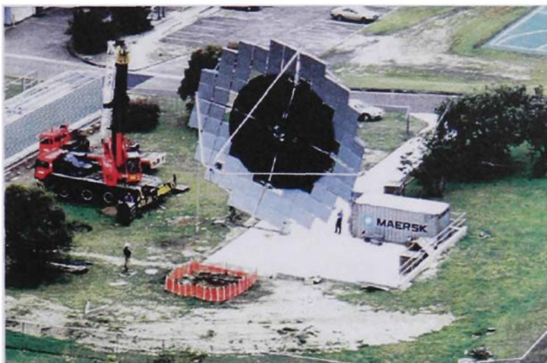
Figure 8-8: Hydrogen Dish designed and built by the researcher and co-workers for the CSIRO to reform natural gas at 750 deg C to make hydrogen. The black louvers are to regulate the concentrated solar power.
