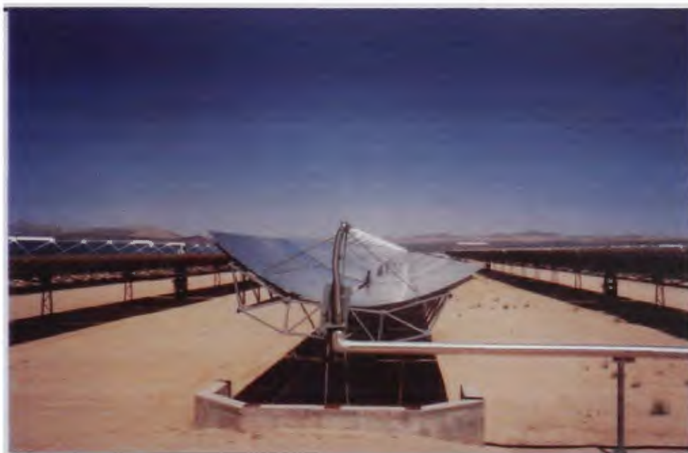
Figure 2-4: Solar thermal trough concentrators at the Solar Energy Generating System (SEGS) plant in California, USA (photo taken by JB Lasich, 1996).
