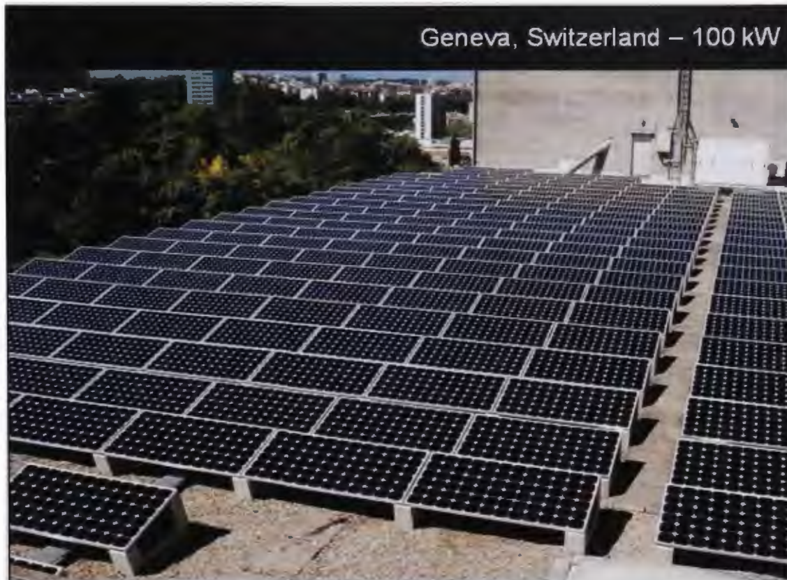
Figure 2-2: A typical ‘flat plate’ installation showing a fixed array of solar panels. The ‘system’ efficiency is typically 8% to 10%, sunlight to AC power, allowing for series mismatch, wiring loss and increase cell temperature.
