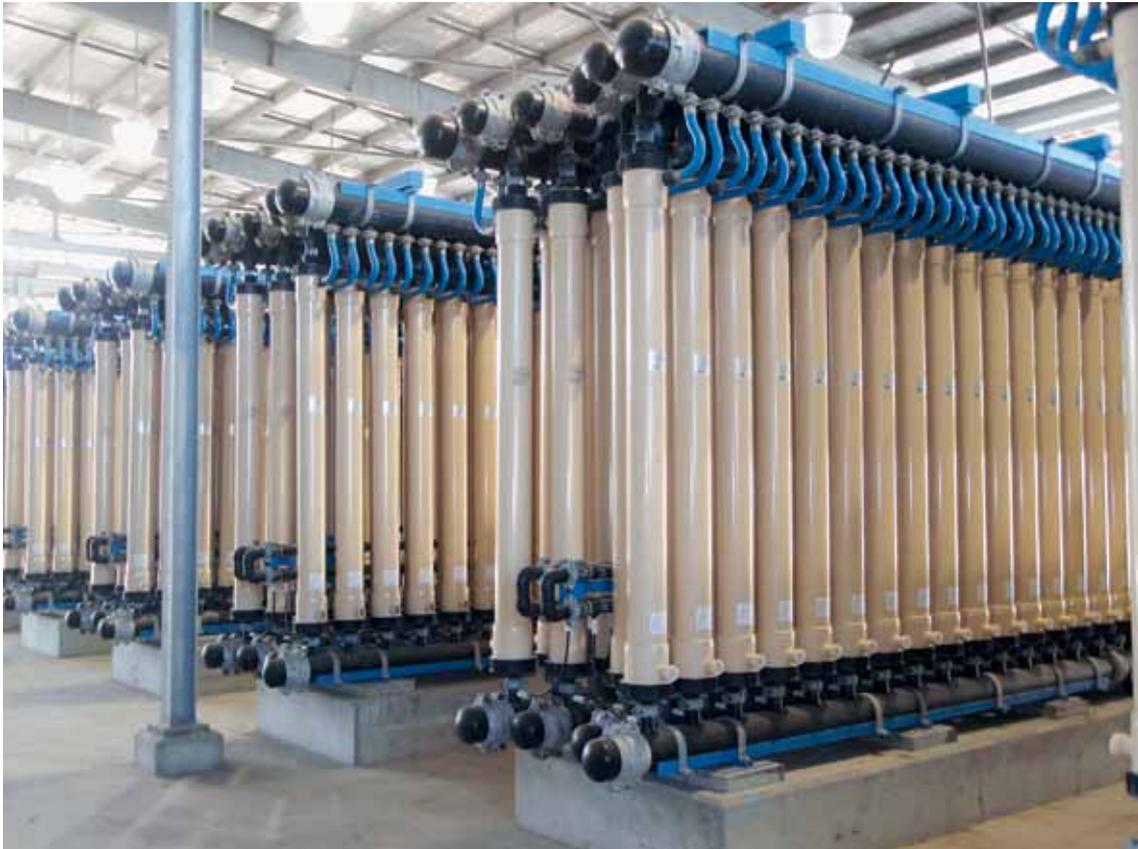
accumulated solids are removed from the surface by a backwash. In the cross-flow process, the feed stream is pumped across the membrane surface which establishes a velocity gradient with a minimum at the membrane surface. A variety of mechanisms including inertial lift and shear enhanced diffusion facilitate the transport of retained material away from the membrane and out of the module.
