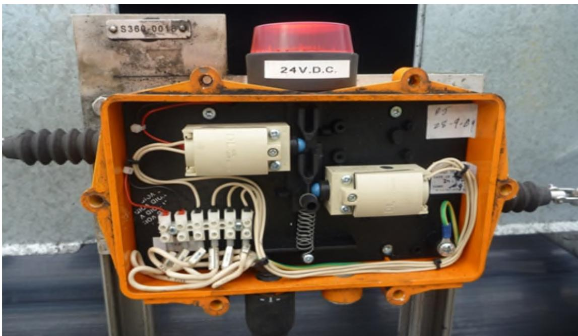
**Fig. 3.5.** SIF#1 (A100) - Safety Switches
