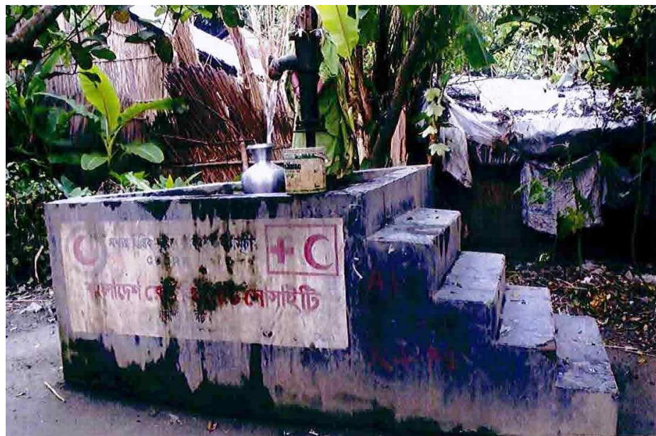
Figure 4.10: Elevated tube well (author’s photo)
