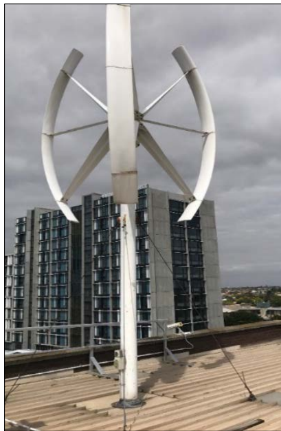
Figure 7.15 3kW rated Wind turbine on the rooftop of Building D at VU, Footscray, Australia
