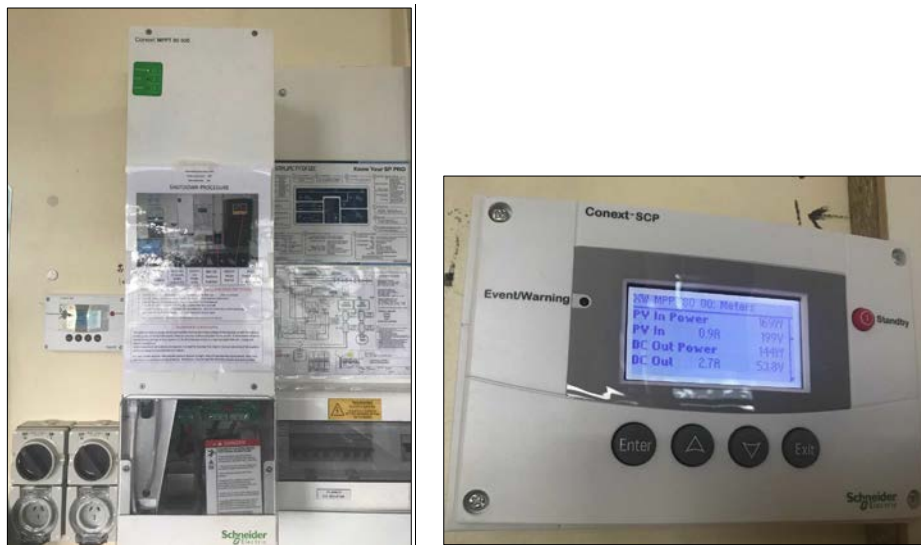
Figure 7.16 (a) and (b) Conext MPPT 80 600 solar charge controller and the display screen
