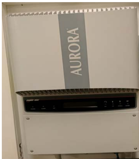
Figure 7.5 Inverter connected to a WT (Aurora PVI 3.6-Outd-AU-W)
