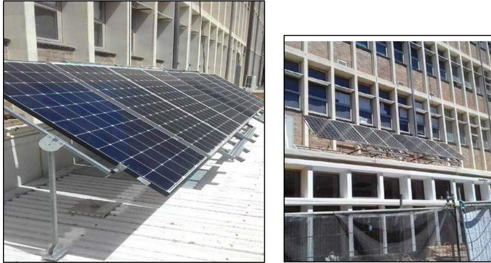
Figure 7.14 (a) and (b) The newly upgraded set of PV panels installed along with the pre-existing PV panels
