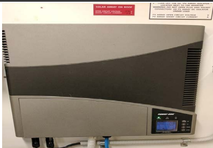
Figure 7.4 Inverter connected to PV modules (Aurora PVI-2000AU)
