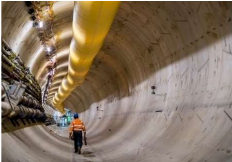
Figure 4 - Melbourne's Metro Tunnel construction with a TBM with reinforced concrete shield lining, Located in Melbourne, Victoria, Australia [11]
