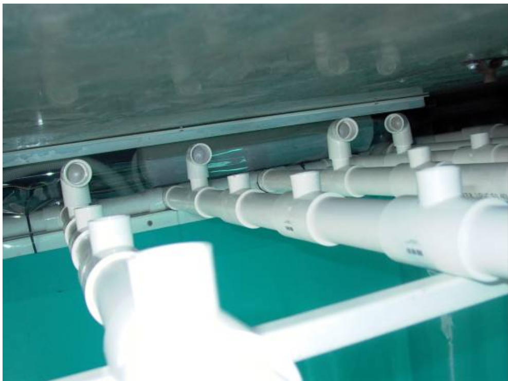
Figure 3.5. A view of the water distribution system in the roof of the shipping container. Water puthers out of the upwards-facing tee-pieces. The inwards facing bends at the rear of the photograph help to ensure that the water is directed towards the produce.
