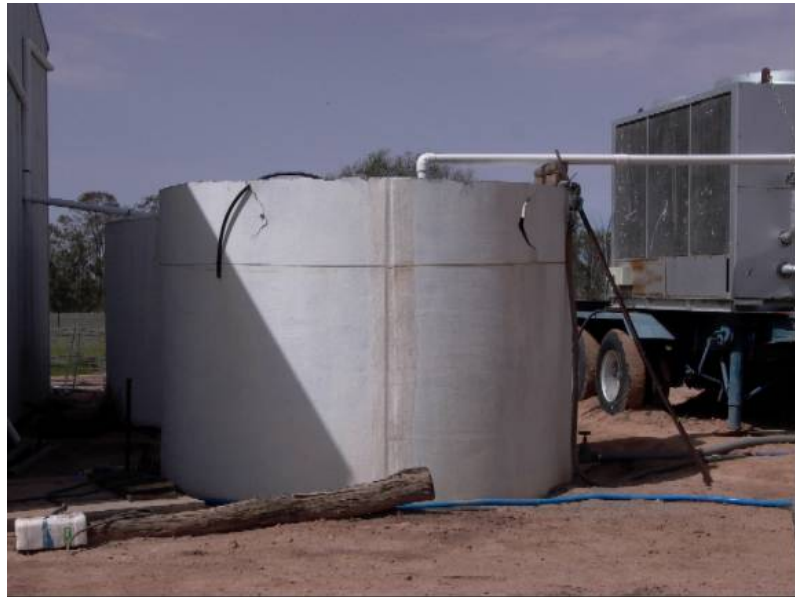
Figure 5.5. The tank used to store chilled water when the cooling unit was located at a property in Goondiwindi, Queensland. The pipe leading from the chilling unit can be seen replenishing the tank. The blue hose on the ground leads to the hydrocooler.
