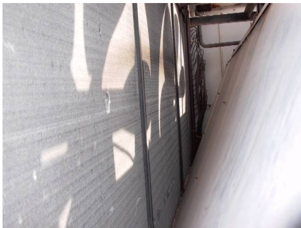
Figure 5.4 The finned coils on the left hand side of the photograph constitute the condenser of the water chilling unit.
