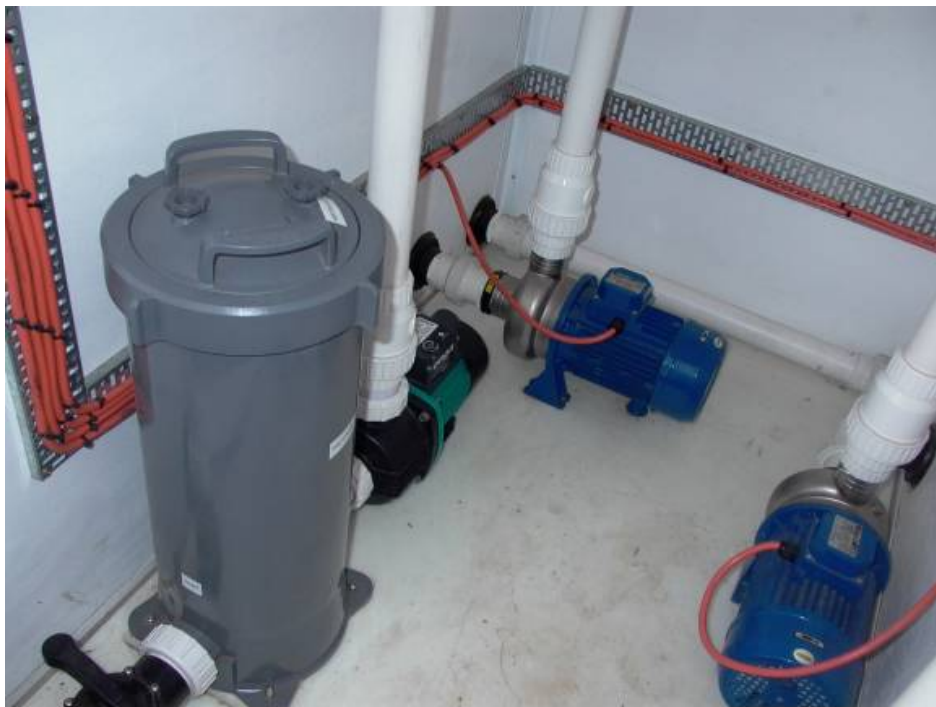
Figure 3.13. The pump room located between bays 2 and 3. Water from bay 2 is strained before being pumped by the green Onga pump to tanks 5 and 6. The blue Ebara pump near the centre of the figure pumps water from the reservoir of Bay 2 to the water distribution system that is located above Bay 2.
