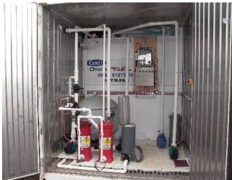
Figure 3.11. The general layout of the filter room showing the blue Ebara DW 400 pump that is used to pump water from bay 1 to one of the water distribution arrays. The green Onga pump draws water from bay 1 whence it is strained and distributes it to tank 2 thus promoting mixing. The photograph shows the stainless steel strainer in the filtration and chemical dosing system removed from its housing. Water leaving this strainer is pumped by an Onga pump to the sand filter – the grey, almost spherical component on the left of the figure. The cylinders that contain the disinfectant, bromo-chloro-dimethylhydantoin, are red.
