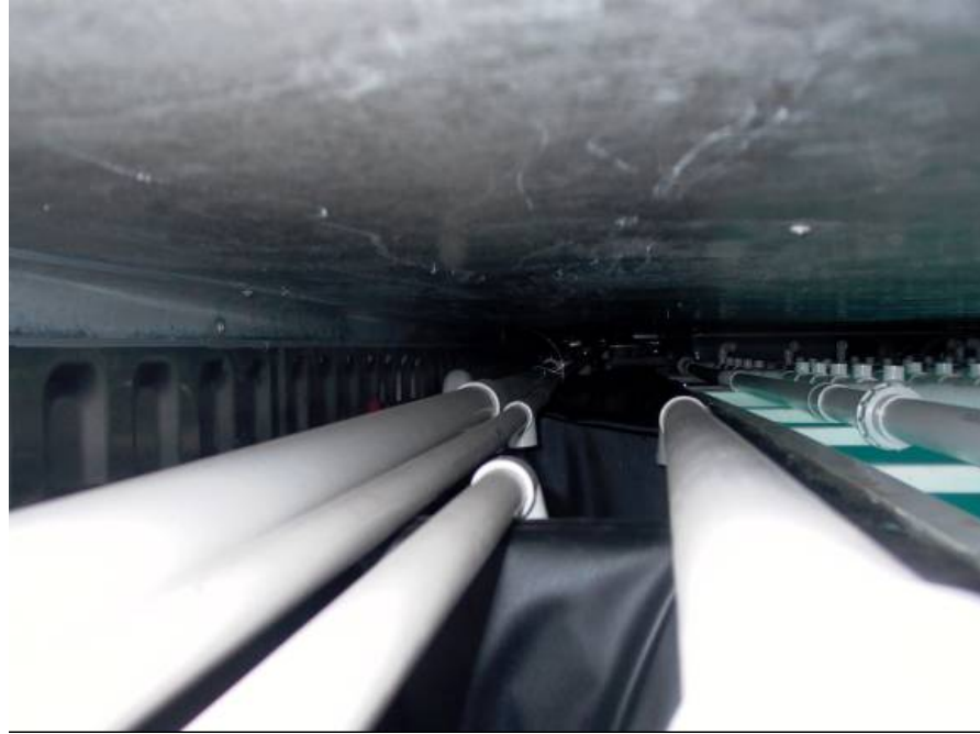
Figure 3.14. Pipes carrying chemically dosed, filtered and water from Bay 1 to the water tanks located at the rear of the hydrocooler. The pipes are laid over the water tanks located at the rear of the hydrocooler.
